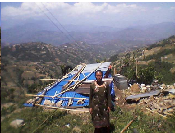
A tin hut as shelter
